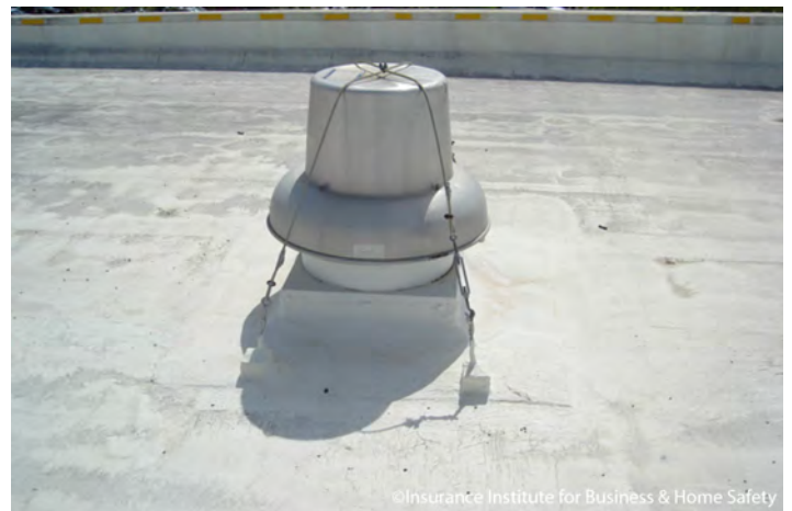
Don't leave roof-mounted HVAC systems exposed to severe weather without proper protection.
