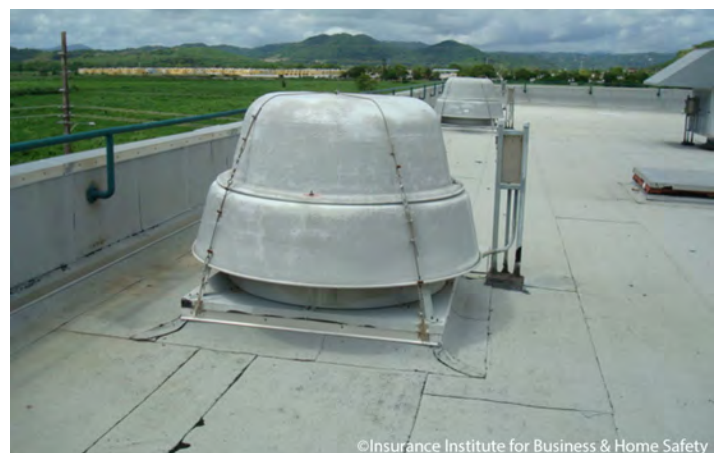
Is your business located in a high wind-prone area? Reinforce roof-mounted equipment with stainless steel cables and turnbuckles (shown above) to reduce risks.
