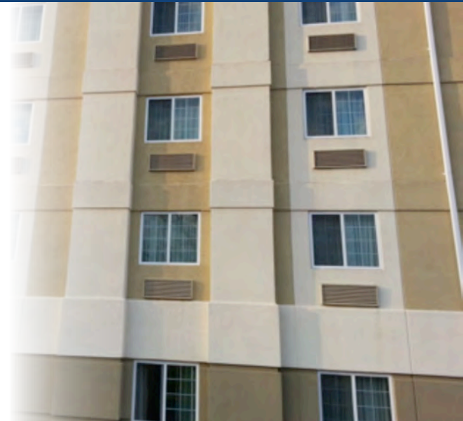
Typical hotel with Exterior Insulating Finishing System.
