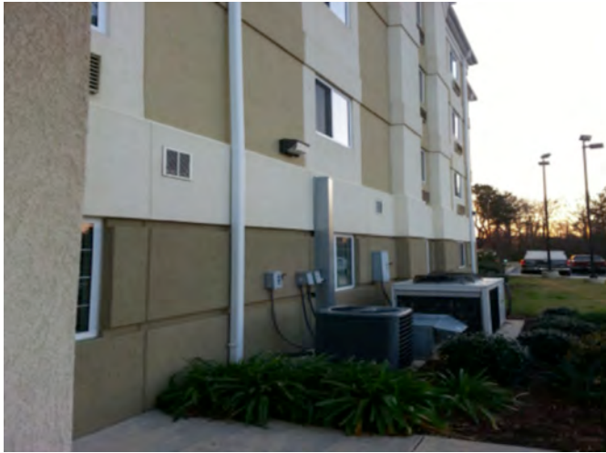
EIFS with multiple corners, edges, windows, joints, penetrations, and wall-mounted AC units.
