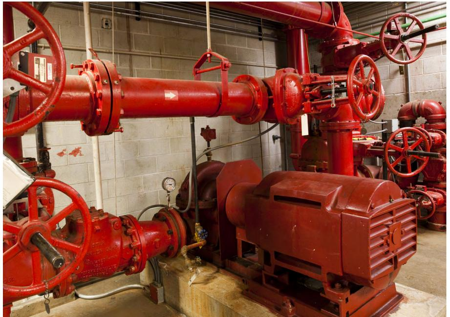
The reliable operation of fire pumps is critical to your fire protection system. They deliver the flow and pressure required for your sprinkler system to respond to a fire. As with any mechanical system, preventive testing and maintenance are needed to ensure the pump operates when it's needed to help protect your business from a catastrophe.
