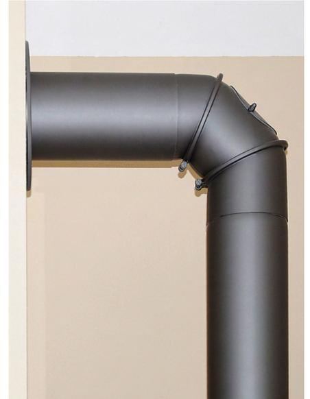
The venting system consists of lengths of 24-gauge or heavier stovepipe that connect the stove to the chimney.
